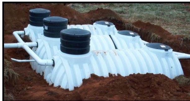
Fig. 8: Below ground tank
