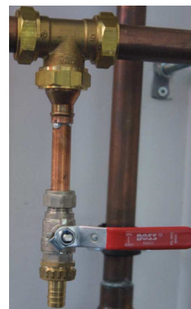
Monitoring equipment for the RWH system - meters (left) and water quality sampling point (right)
