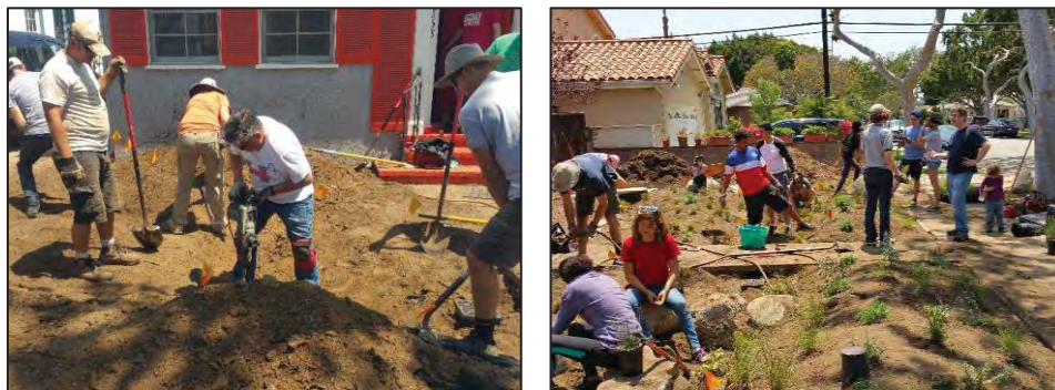
Figure 12. Volunteers helping install a rain garden: preparing the bioswale (left); plant vegetation (right) (May 2016).
