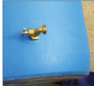
Figure 18. Hose bib facing to the side.
