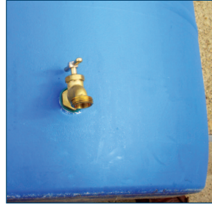
Figure 17. Hose bib facing down.
